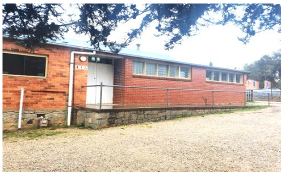
Figure 5: West side of the hall – access ramp
