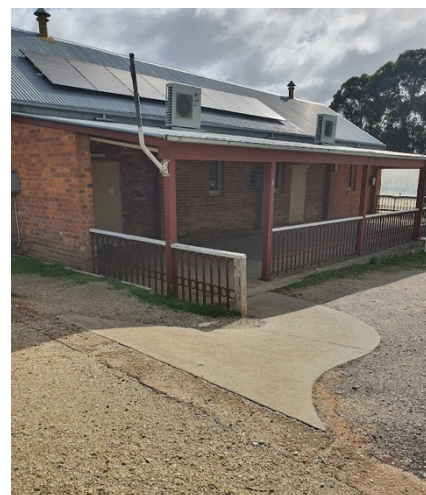
Figure 25: Access path into hall from Duke St.
